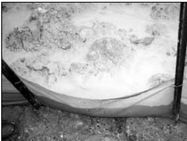
Figure 2.11 A geotextile fence used to trap fine sediment generated from a construction site
