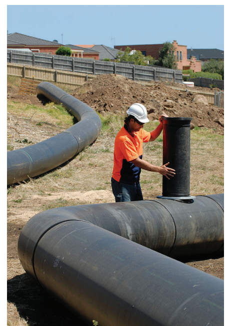
Inspecting the “inspection opening” on the trunk pipeline before laying.
