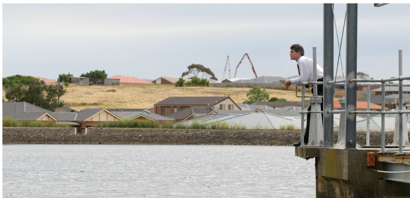
Peter Wilson looking over the Brierly Raw Water Basin, receiving storage for harvested roof water. The tiled roofs seen in the background are connected to the system.
