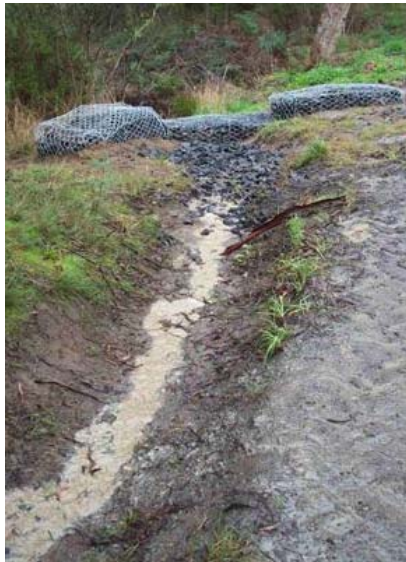
Photo 10: A sediment trap constructed from gabions.
