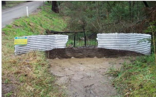
Photo 11: A sediment filter used to construct a sediment trap.
