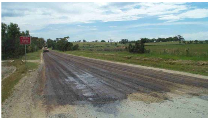
Photo 14: Dust suppression application.
