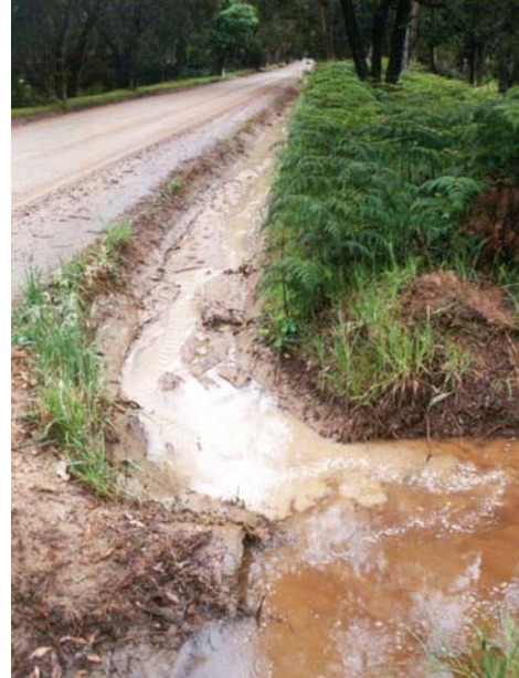
Photo 1: Sediment runoff from an unsealed road.
