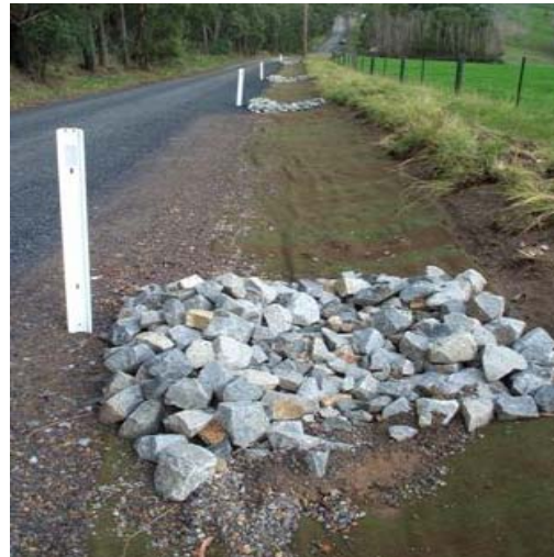
Photo 7: A series of rock check dams.
