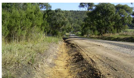
Photo 5: A recently cleaned table drain.
