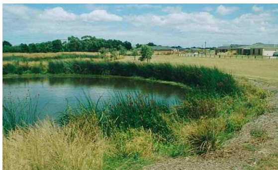
Photo 12: A wetland used to treat stormwater runoff from a subdivision in Officer.
