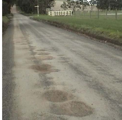
Photo 3: Potholes in an unsealed pavement.
