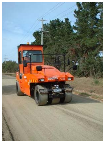
Photo 2: Multi-wheel roller compacting a section of Boes Rd Hastings.
