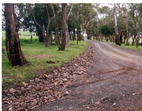
Photo 6: A table drain lined with rock rubble.
