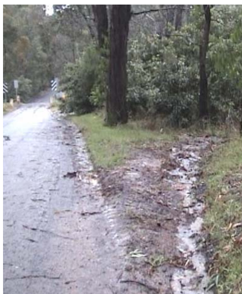
Photo 8: Cut-off drain diverts runoff into a stable vegetated area.
