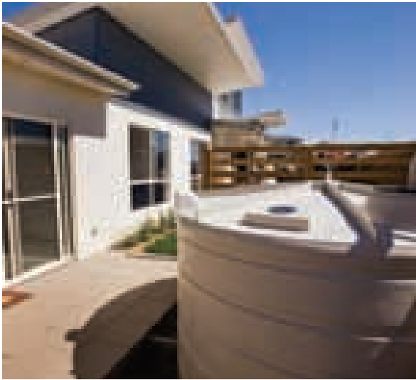
Domestic rainwater tank. Photo: CSIRO.
