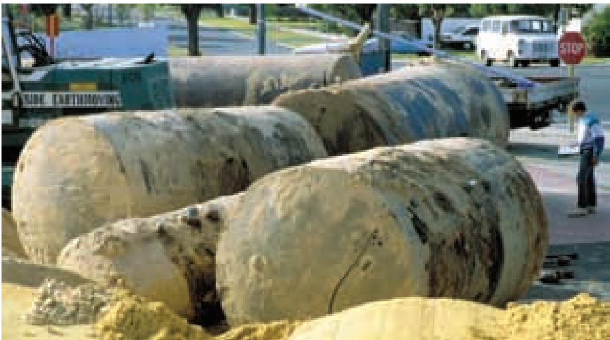
Removal of service station fuel tanks which can leak into groundwater, Perth, Western Australia. Photo: Bill van Aken, CSIRO.
