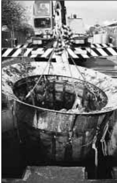
The CRC study included an investigation of cleaning procedures for the CDS device. After cleaning, remaining material was collected and compared to the mass removed. The study revealed that a vacuum cleaning method is best suited to the Coburg installation.
