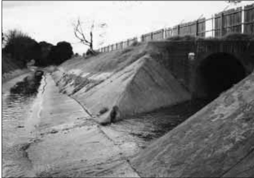
*Concrete-lined drains transport pollutants efficiently*
