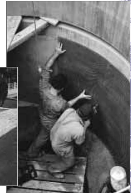
*Construction of the CDS device (clockwise from top left): digging the hole for construction; walls of the collection chamber; fitting the separation screen; and the final product at road level*
