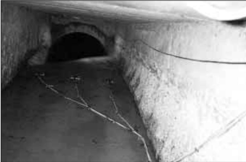
*CDS instrumentation included depth probes (above) and flow meters (below)*
