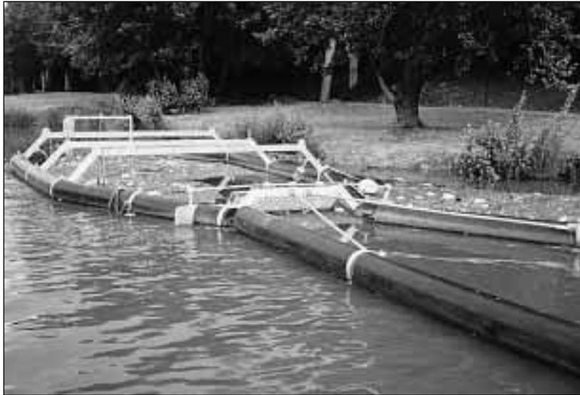
*Floating debris trap in the Yarra River, Melbourne*
