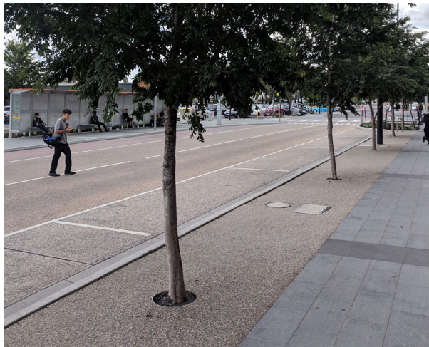
Permeable pavement &amp; structural soil
