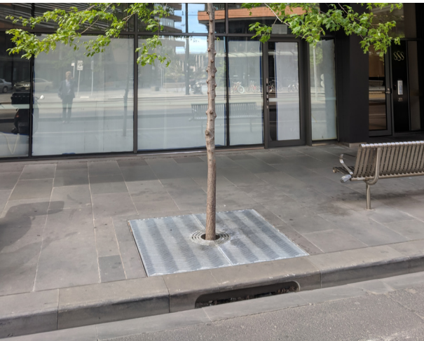
Grated tree pits
