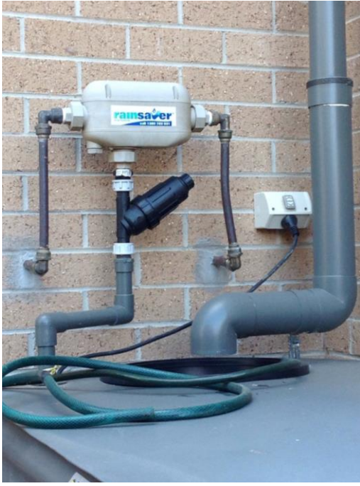
Figure 11: Electronic diverter and in-tank sump-pump with filter.
