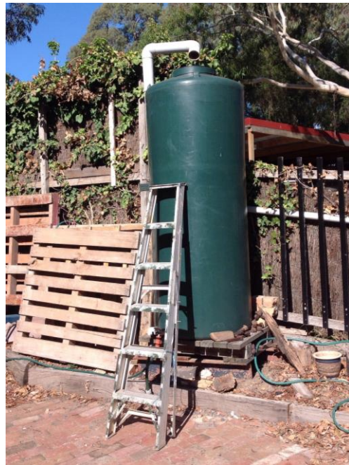
Figure 10: High-risk set-up. High center of gravity, non-concrete base, pallets and ladder at risk of falling, hose is a tripping hazard.
