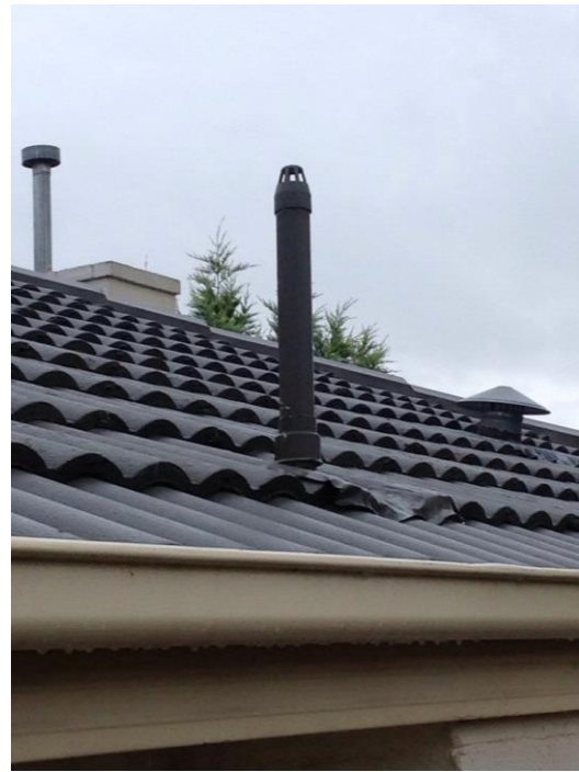
Figure 5: Lead flashing used on air vents.
