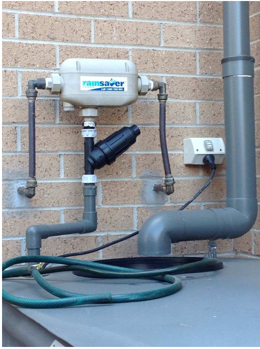
Figure 11: Electronic diverter and in-tank sump-pump with filter.
