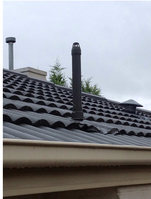
Figure 5: Lead flashing used on air vents.
