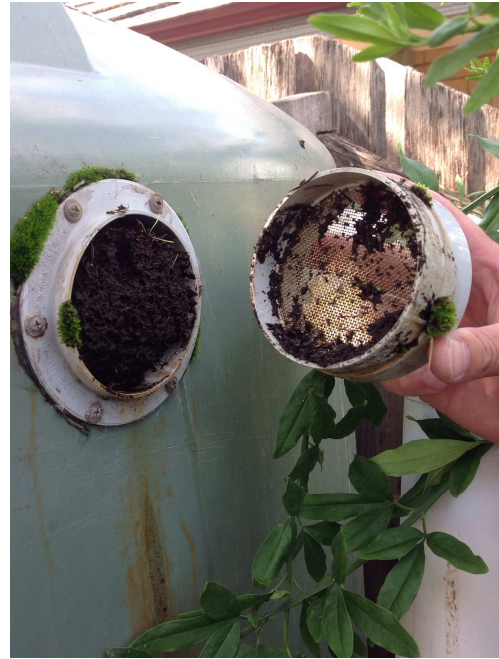
Figure 9: Fouled mosquito mesh at overflow which indicates high levels of sediment in the tank water.
