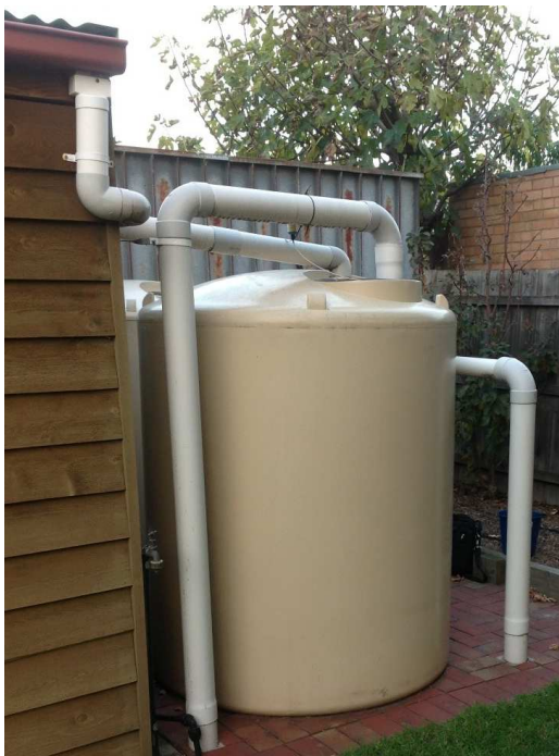
Figure 4: Polycarbonate tank with direct downpipe inflow and wet charge system. Tank installed on pre-existing paving.
