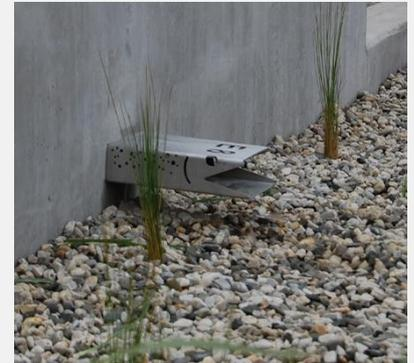
*Stainless steel eel-head spout directs stormwater into the raingardens*
