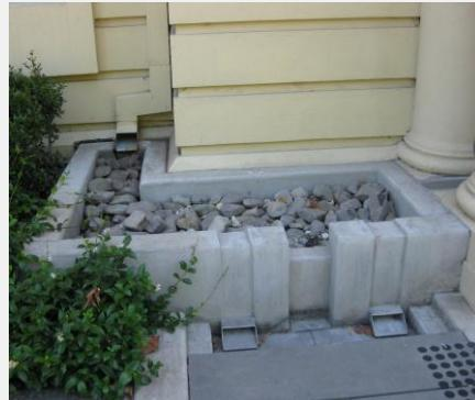
Prior to entering the raingardens, roofwater is directed into a small detention system to reduce flow velocities
