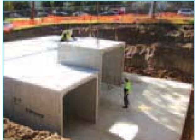
Concrete storage tank under construction using Humes precast components
