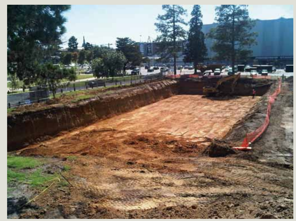
The excavation was 4.5m deep , 65m long and 25m wide
